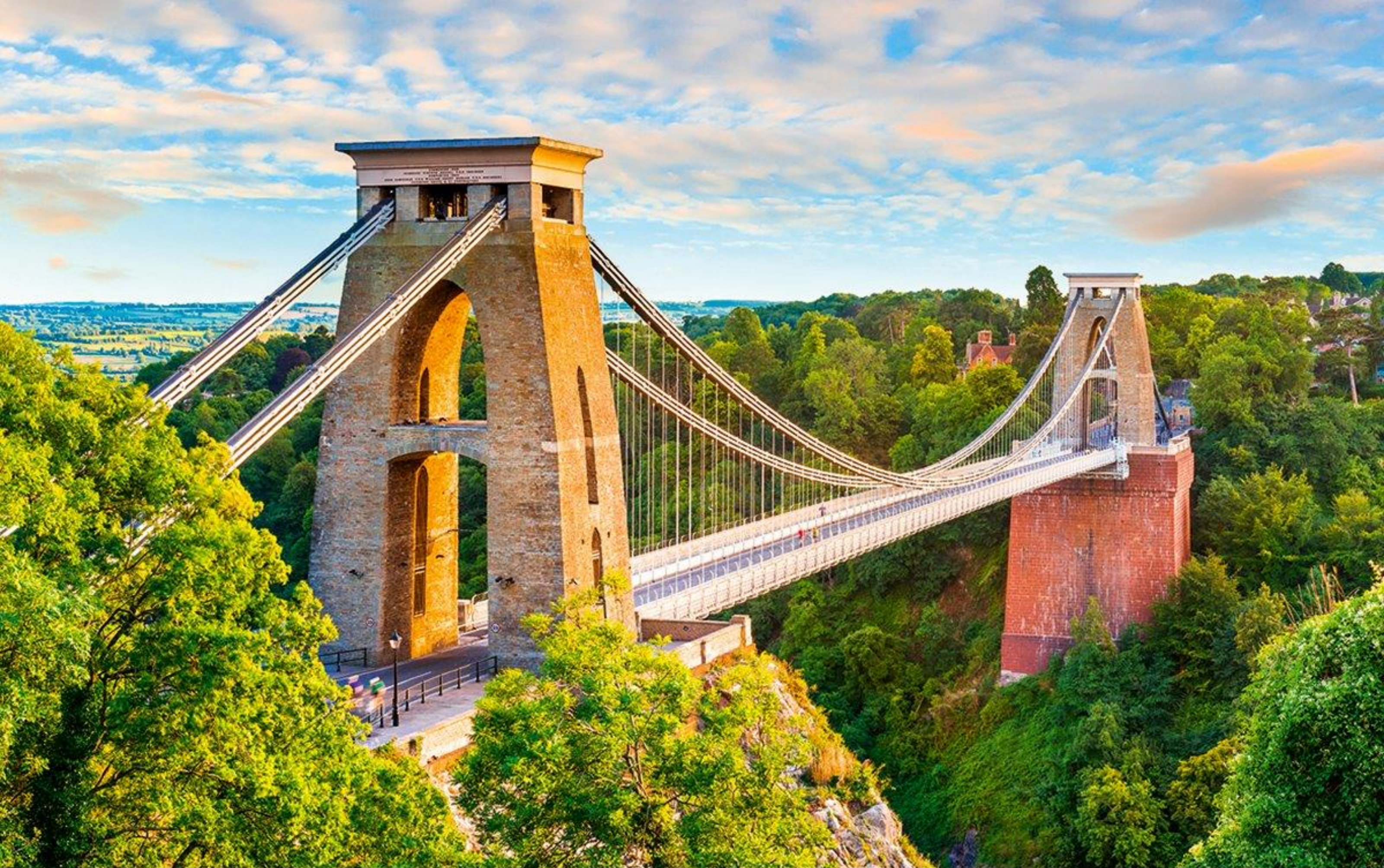
Clifton Suspension Bridge, Bristol, UK. / © Gettyimages
